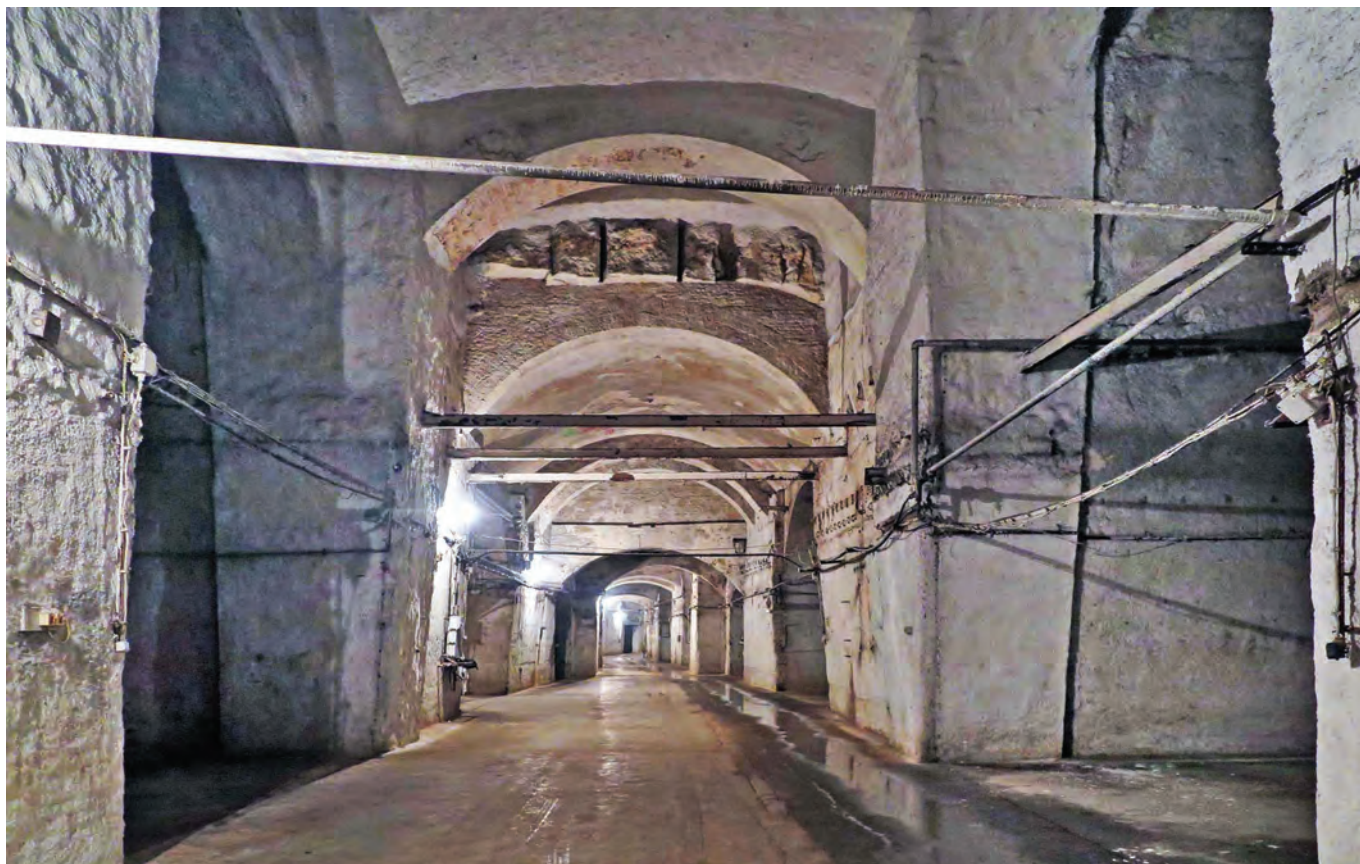
Kőbánya quarry. The ceilings of the original quarry were reinforced by arching and steelwork when it was converted into a brewery
